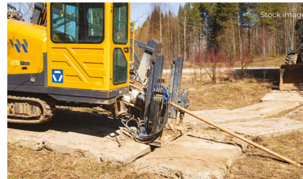
Horizontal Directional Drilling (HDD)
